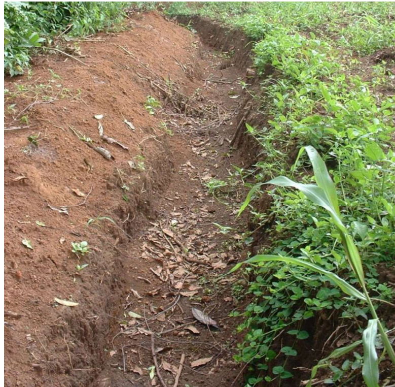
Figure 11 Partially completed trench in Year 2. On completion the trench was twice as deep and the (left) wall close to the forest was much steeper.
