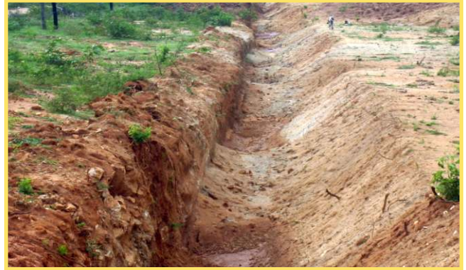
Eroded elephant ditch (newly constructed and abandoned trench), Lunugamvehera National Park Sri Lanka. © Prithviraj Fernando.
