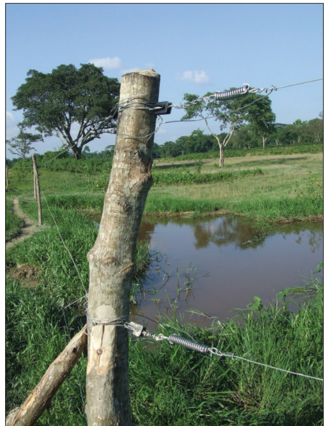
Figure 4. A two-strand electric fence installed in Sonitpur district.
